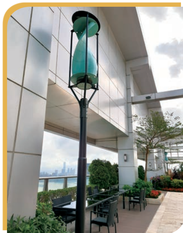
In 2019, BEA installed a self-sustaining outdoor lighting system powered by wind turbines at BEA Tower.
